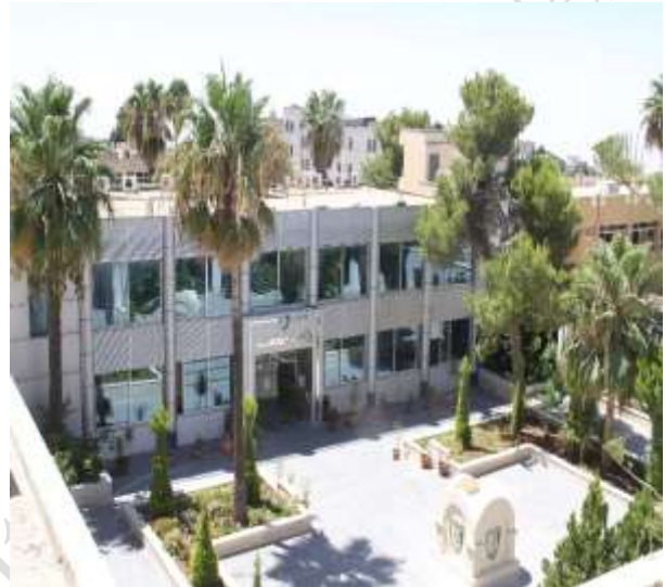
Metal cladding systems
